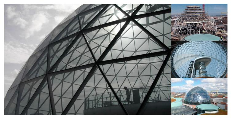
The dome in Victoria Square is part of a shopping centre Project which is being developed in Belfast, Northern Ireland. It is a single-layer dome conceived by LANIK and commissioned by SPACEDECKS LTD., which responds to a spatial structure formed by a series of triangles composed of diagonal and parallel beams.
